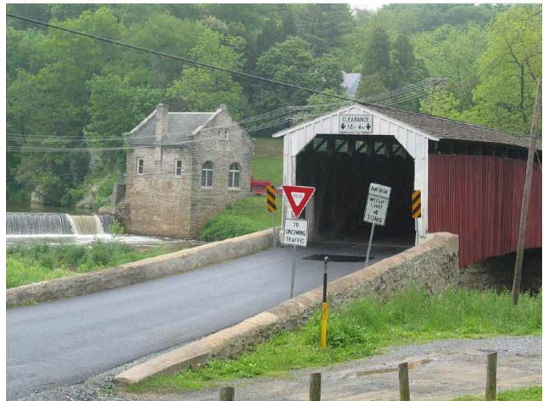
Pine Grove Covered Bridge; pump house studio in background
